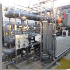
Provided design, specification, permitting, fabrication, manufacturing, installation and certification of wastewater treatment systems for this solar cell manufacturing facility. The treatment included wastewater equalization, pump stations, microfiltration and sludge processing systems.
