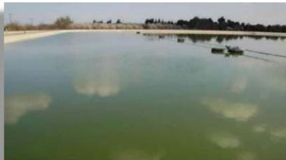
The Hilmar WWT plant has operated since 2004 without accumulating or removing sludge, and Hilmar residents enjoy some of the lowest rates in the state of California. This facility's design includes some of the latest improvements to the Advanced Integrated Pond Systems approach, affording greater energy efficiency and superior process control.
