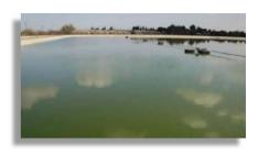
The Hilmar WWT plant has operated since 2004 without accumulating or removing sludge, and Hilmar residents enjoy some of the lowest rates in the state of California. This facility's design includes some of the latest improvements to the Advanced Integrated Pond Systems approach, affording greater energy efficiency and superior process control.
