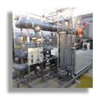
Provided design, specification, permitting, fabrication, manufacturing, installation and certification of wastewater treatment systems for this solar cell manufacturing facility. The treatment included wastewater equalization, pump stations, microfiltration and sludge processing systems.
